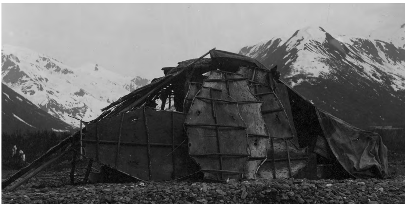
FIGURE 46. Bark-covered smokehouse at Keik'uliyáa sealing camp in Disenchantment Bay. The pole-framed structure is roofed with spruce bark; harbor seal skins stretched on frames have been placed on the roof and against the front. Photograph by Edward S. Curtis, Harriman Alaska Expedition, June 1899. National Museum of the American Indian, Smithsonian Institution P10972.
