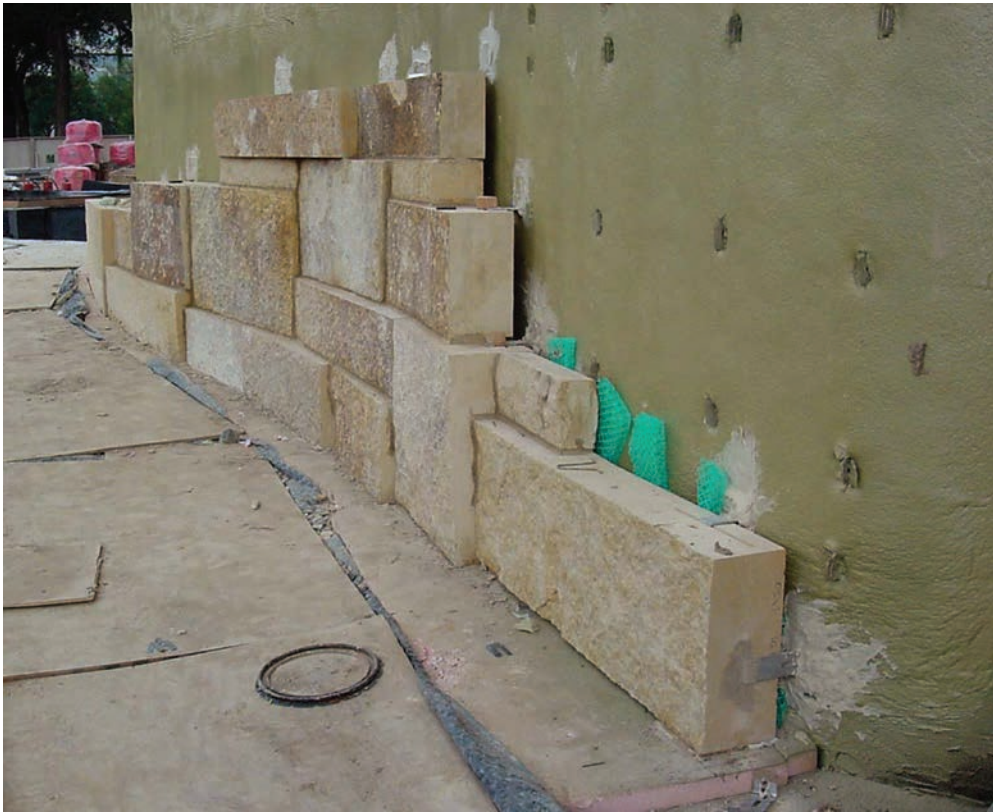
FIGURE 12. Blocks of roughback stone at the base of the building during installation. Note the stainless-steel brackets that secure each stone at the sides and on top to the interior structure. Photo by Michael Dobbs, SmithGroup.
