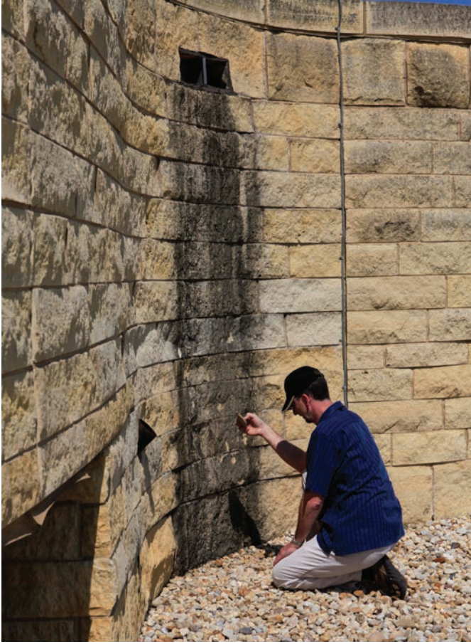
FIGURE 19. Light-colored spots in the thick, dark deposit under a scupper, detail of Figure 18, showing detachment and flaking of the stone in 2010. Photo by E. Keats Webb, Smithsonian Institution.
