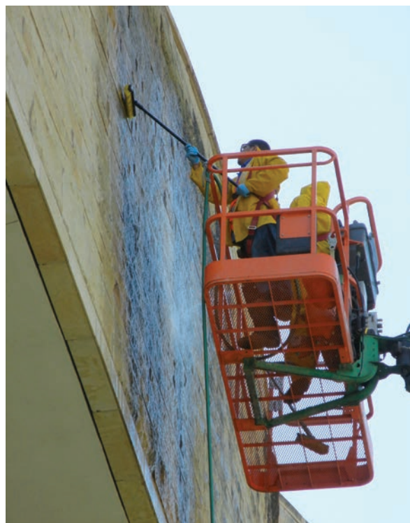
FIGURE 7. Application of the biocide D/2 to the most severely streaked area below the Inouye Terrace (left), followed by scrubbing the area (right) on April 15, 2011. Photo by Carol A. Grissom, Smithsonian Institution.
