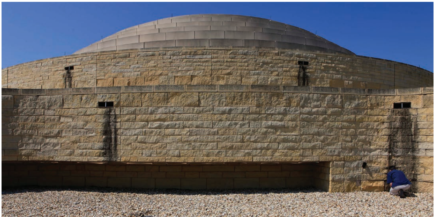
FIGURE 18. Thick, dark deposits under scuppers (type F) that drain roofs atop the NMAI building with flows of large amounts of water in 2010. Photo by E. Keats Webb, Smithsonian Institution.
