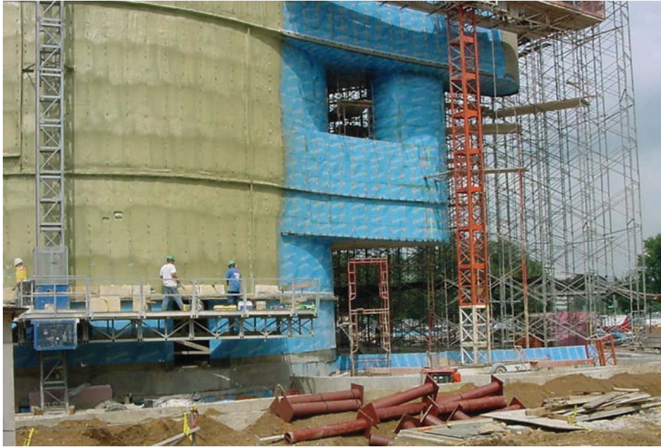
FIGURE 9. Installation of splitface blocks at the southeast corner of the building. Note the blueskin moisture barrier, brown polyurethane foam, and shelf brackets at horizontal intervals. Photo by Michael Dobbs, SmithGroup.
