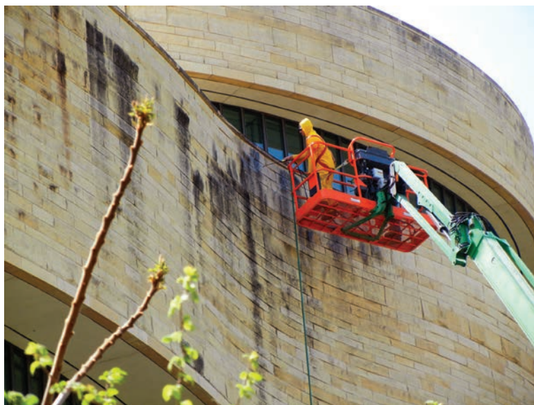
FIGURE 7. Application of the biocide D/2 to the most severely streaked area below the Inouye Terrace (left), followed by scrubbing the area (right) on April 15, 2011. Photo by Carol A. Grissom, Smithsonian Institution.
