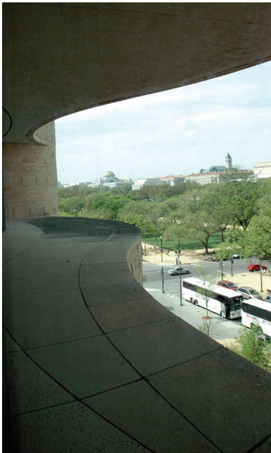
FIGURE 11. Dark deposits at the unprotected end of the deck of north facade balcony 2, seen from the fourth floor inside the museum, in 2010. Dark streaks occurred on the facade below, although the outermost stones slope inward on this balcony. Photo by Carol A. Grissom, Smithsonian Institution.
