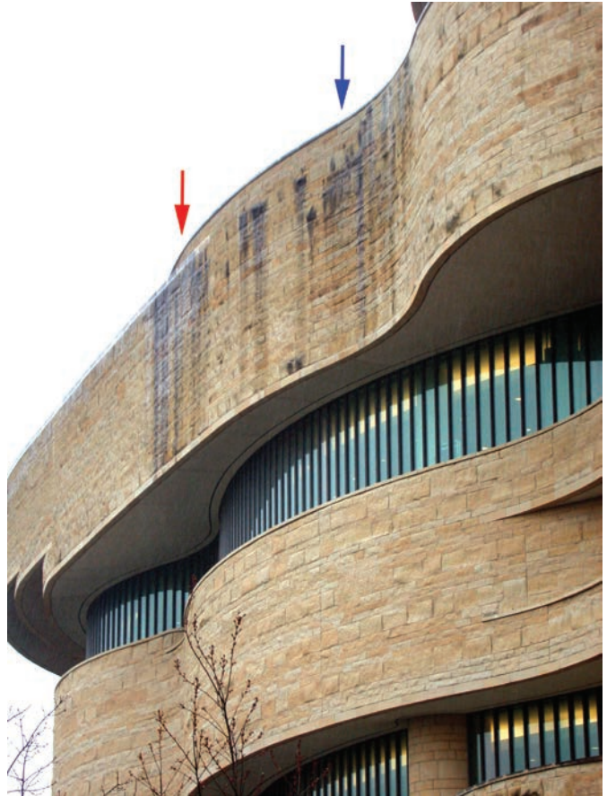
FIGURE 16. (Left) Wetting of the area shown in Figure 15, photographed during a rain event in 2010; arrows are as in Figure 15. Photo by Carol A. Grissom, Smithsonian Institution.
