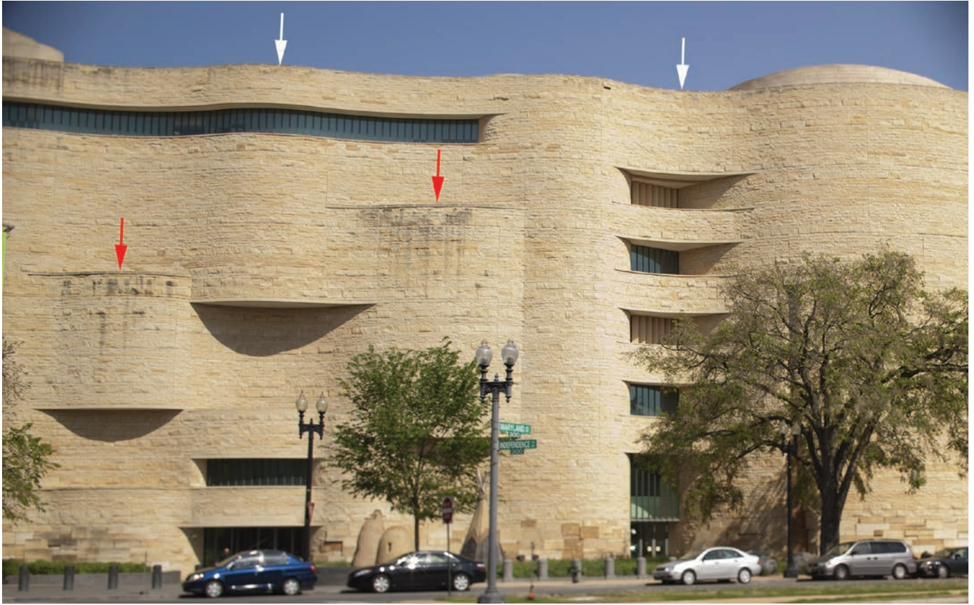
FIGURE 5. Clean-looking stone below balconies protected by overhangs on the south facade (white arrows), in contrast to darkened stone below those that are not protected by overhangs (red arrows), in 2010. Photo by Melvin J. Wachowiak and E. Keats Webb, Smithsonian Institution.
