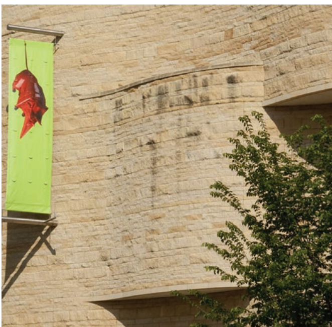
FIGURE 6. Detail of dark streaking (type C) below the unprotected balcony on the left in Figure 5 in 2010. Photo by Melvin J. Wachowiak and E. Keats Webb, Smithsonian Institution.
