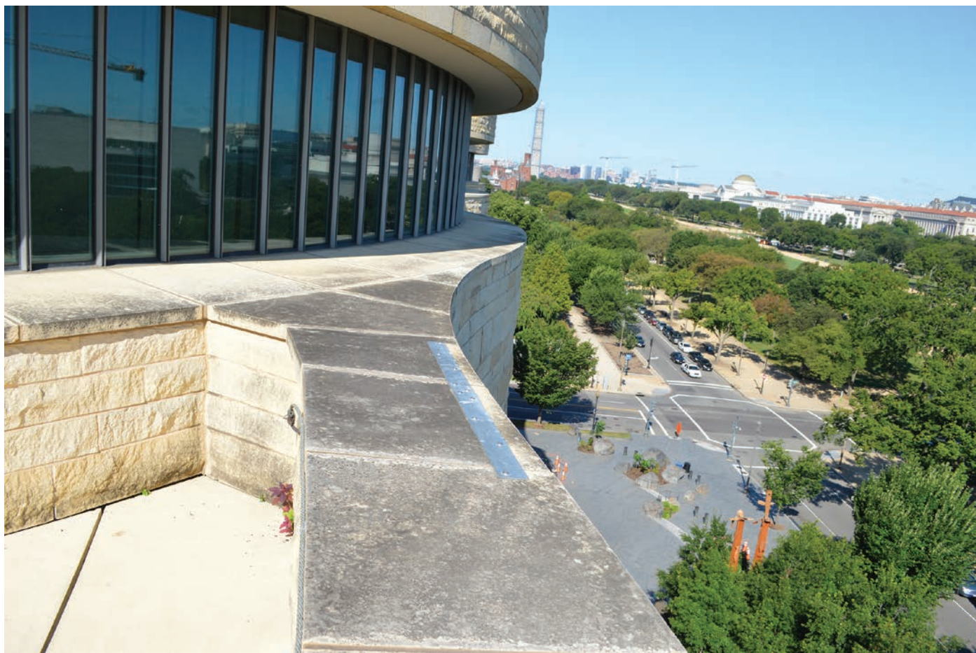
FIGURE 11. Second and third blocks on the Inouye Terrace, to which zinc strips have been attached, shown 18 months after installation on August 14, 2013; see figure 15 of Grissom and Charola (this volume). Photo by Carol A. Grissom, Smithsonian Institution.
