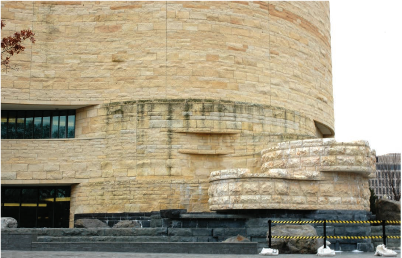
FIGURE 4. Prominent dark streaks (type C) below the balcony's capstone joints above the cascade at the northwest corner in contrast to generalized darkening visible on the sides of capstones in 2010. Photo by Carol A. Grissom, Smithsonian Institution.
