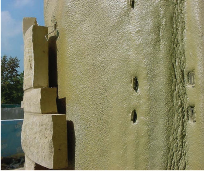
FIGURE 11. Detail showing stainless-steel hardware used to attach the Kasota limestone, west facade. Photo by Michael Dobbs, SmithGroup.
