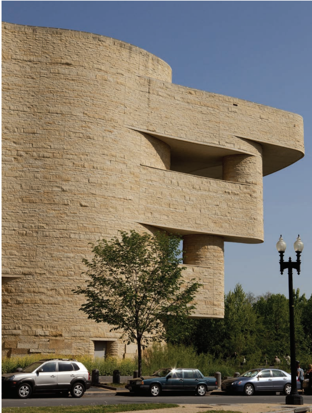
FIGURE 3. Slight, relatively uniform darkening (type B) immediately below the roofline of the south facade in contrast to clean-appearing areas below overhangs at right in 2010. Photo by Melvin J. Wachowiak and E. Keats Webb, Smithsonian Institution.
