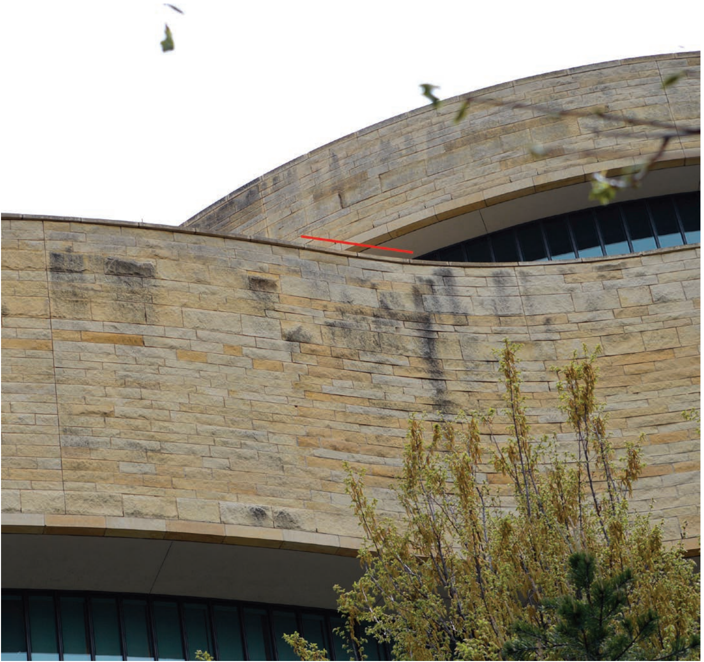
FIGURE 12. Detail of the facade below capstones on which zinc strips shown in Figure 11 were installed (location indicated by the red bar), eight months later (two years and two months after installation). Note that front faces of the blocks were cleaner than surrounding blocks in April 2014. Photo by Carol A. Grissom, Smithsonian Institution.
