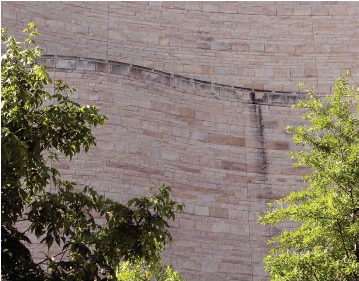
FIGURE 10. Darkening on stonework of the facade below north facade balcony 1, although the capstones slope slightly inward to drains, in 2010. Photo by Melvin J. Wachowiak and E. Keats Webb, Smithsonian Institution.
