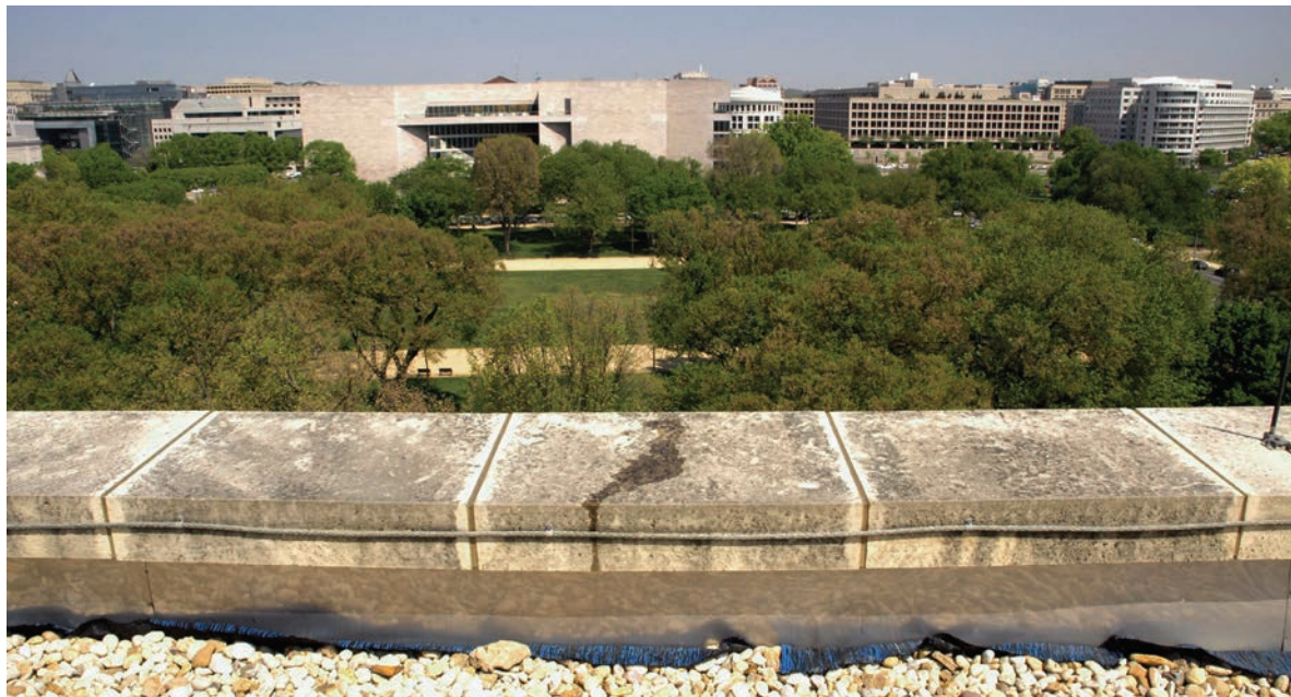
FIGURE 1. Darkening of capstones on the roofline (type A) in 2010. Flow of water in both directions when poured onto the center of the middle stone shows that the stone is essentially level. Note the light areas next to joints where water repellent components of silicone sealants bled into the stone. Photo by Carol A. Grissom, Smithsonian Institution.
