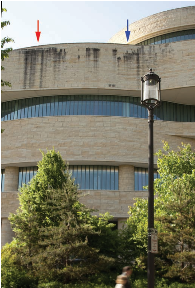
FIGURE 15. Dark streaks on the facade (type E) below the Inouye Terrace on the north facade in 2010. The red arrow indicates streaking compounded by runoff from both the terrace and an intersecting parapet wall. The blue arrow indicates streaking by increased runoff from stones sloping toward the intersection of the window sill and parapet wall. Photo by Melvin J. Wachowiak and E. Keats Webb, Smithsonian Institution.
