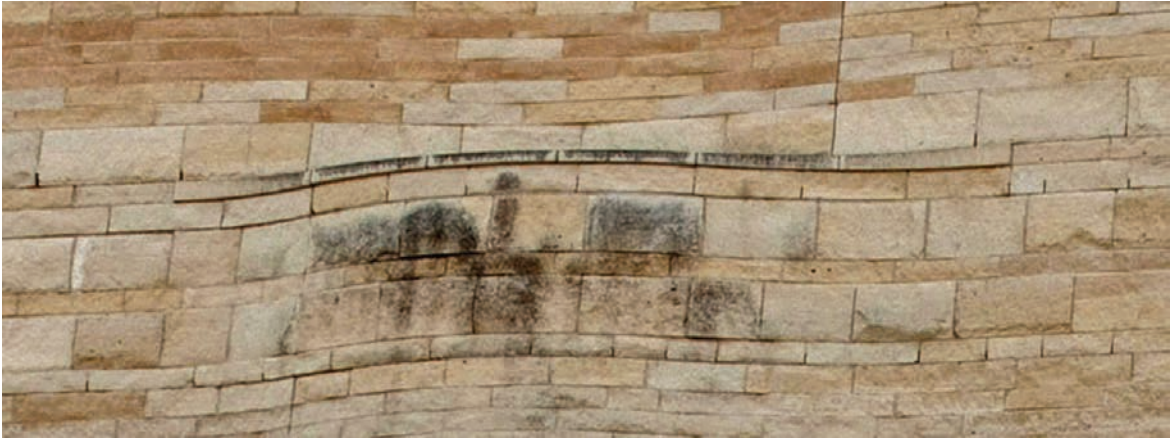
FIGURE 9. Generalized darkening below capstones toward the center of west facade balcony 1, probably from water flowing over the center capstones that are more sloped than those on the sides, in 2010. Photo by Melvin J. Wachowiak and E. Keats Webb, Smithsonian Institution.
