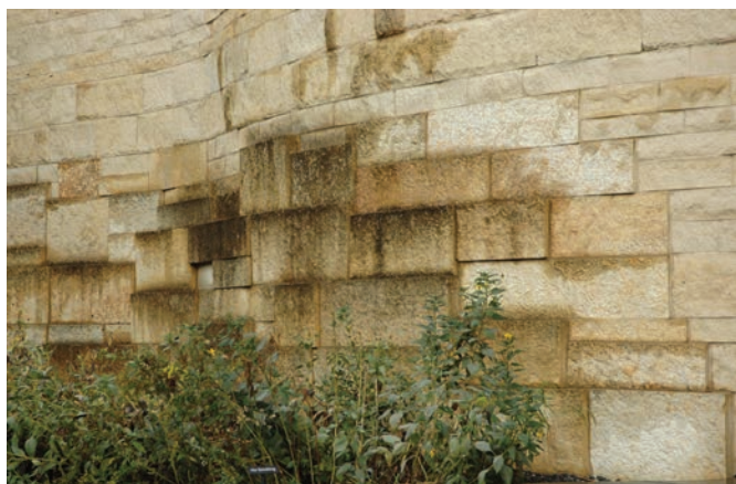
FIGURE 13. Wetting and darkening of other roughback blocks (type D) with shielding vegetation nearby, such as these to the left of the Independence Avenue entrance to the building; photographed just after a rain event in 2010. Photo by Carol A. Grissom, Smithsonian Institution.
