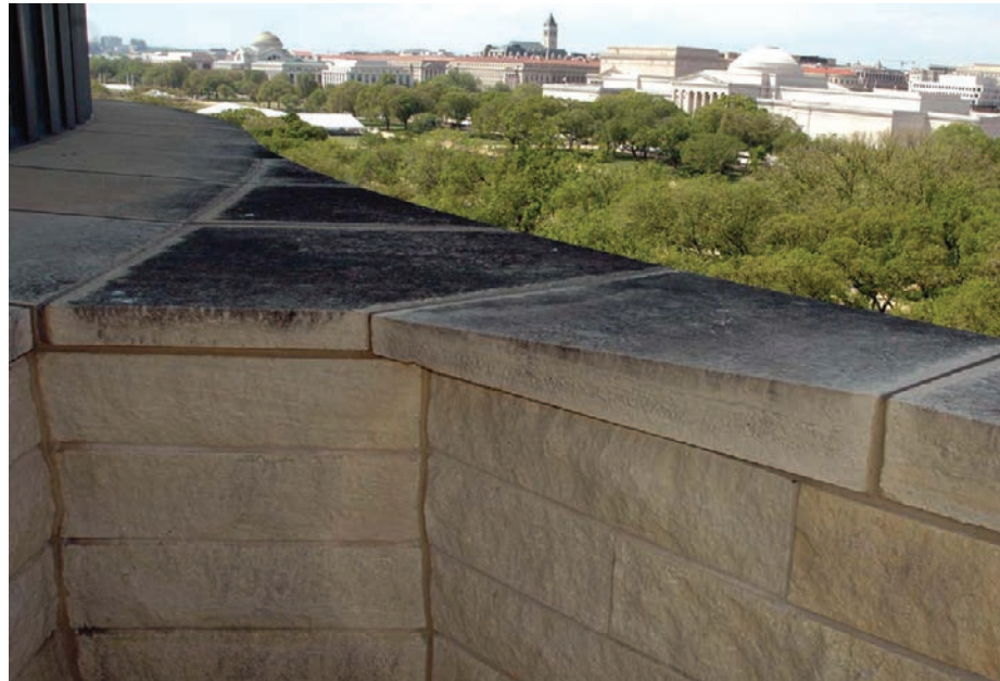
FIGURE 17. Darkening of capstones at the intersection of the Inouye Terrace parapet wall with the windowsill on the left in 2010. The large capstone displaying the darkest surface on the left slopes down and outward, whereas the stone to its right slopes toward it. During rainfall a large volume of water is funneled over these capstones onto the facade, contributing to the severe dark streaks seen in Figures 15 and 16. Photo by Carol A. Grissom, Smithsonian Institution.
