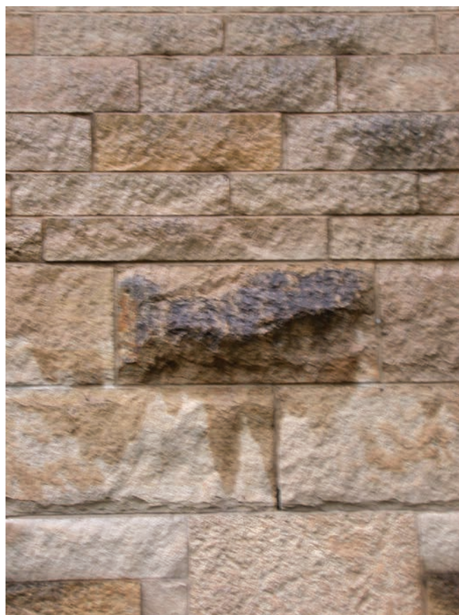
FIGURE 14. Wetting and darkening of the protruding block at the center (type D), photographed just after a rain event in 2010. Photo by Carol A. Grissom, Smithsonian Institution.
