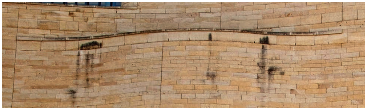
FIGURE 8. Dark streaking below a few capstone joints on west facade balcony 2 in 2010. Photo by Melvin J. Wachowiak and E. Keats Webb, Smithsonian Institution.
