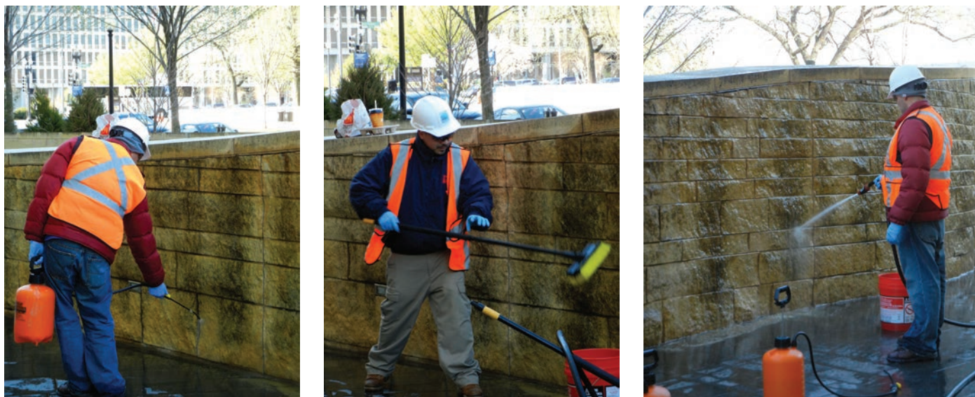
FIGURE 5. Application of D/2 on the loading dock wall (left), followed by scrubbing (middle) and rinsing with water (right) on April 6, 2011. Photo by Carol A. Grissom, Smithsonian Institution.
