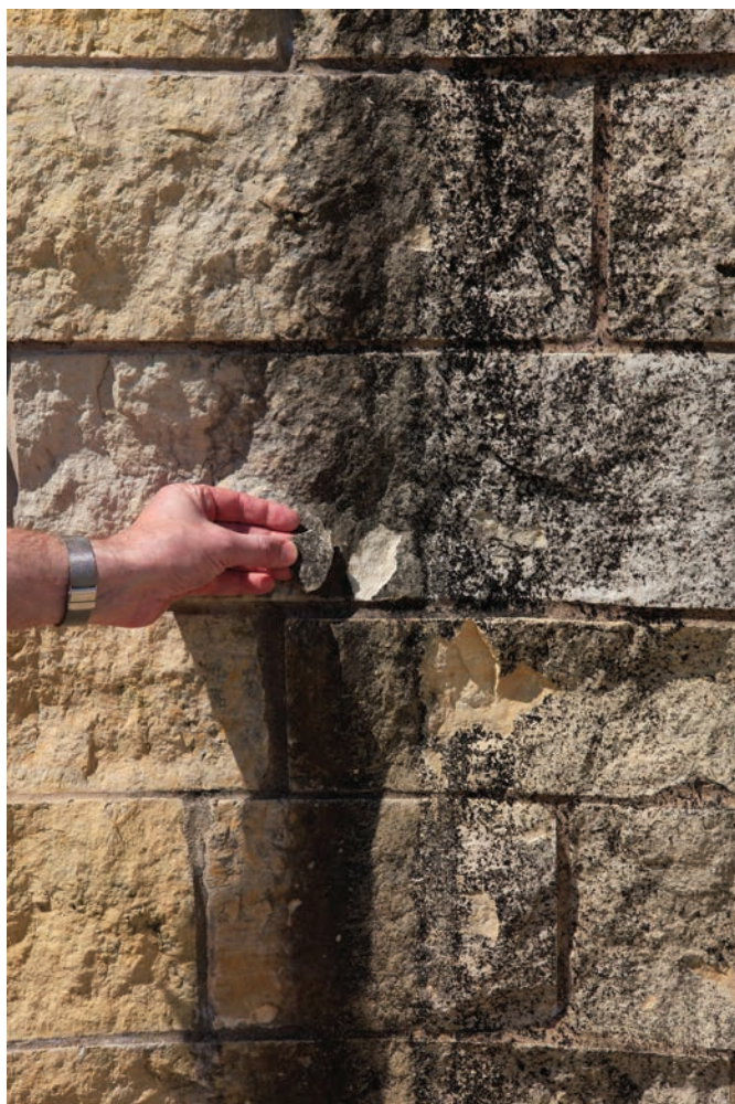
FIGURE 3. Exfoliation of the Kasota limestone from the NMAI building in the area below a scupper water drain on the east terrace wall beyond the Senator Inouye Terrace (see figure 18 in Grissom and Charola, “Survey and Documentation of Darkening and Streaking on the National Museum of the American Indian Building,” this volume). The exfoliation or spalling is potentially a result of the blackish epilithic colonization.
