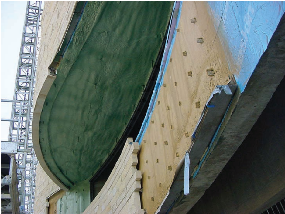
FIGURE 10. North wall layers visible during construction: (from interior) concrete structural masonry, blueskin barrier, stainless-steel hardware at intervals with brown foam insulation over top, a 5-cm-wide air gap, and Kasota limestone. A shelf bracket is visible at the base of the brown foam insulated area. Photo by Michael Dobbs, SmithGroup.
