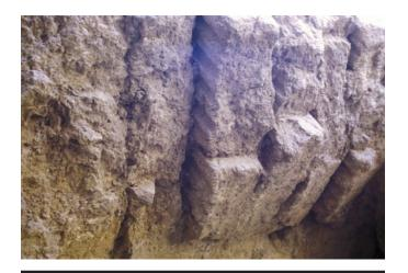
FIGURE 8.166. Square 1A: mortar between grooved bricks in a vault.
