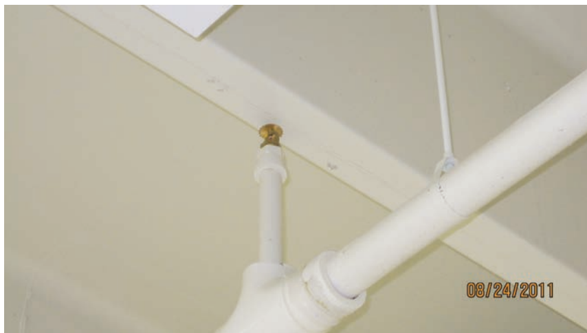
FIGURE 3. Above, sprinkler head as installed; right, sprinkler head in Pod 3 sheared off during the earthquake. (Smithsonian Institution photo by Catharine Hawks, NMNH.)
