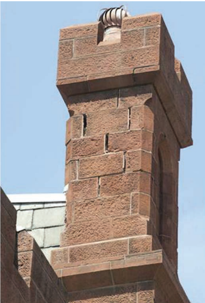
FIGURE 11. The Smithsonian Castle (above) and damage that some of the towers suffered as illustrated by the displacement of blocks in the chimney (detail, left). These blocks are high-quality Seneca sandstone and each one weighs some 68 kg (150 lb). (Smithsonian Institution photos: Castle, Donald E. Hurlbert; chimney detail, Mark Avino.)
