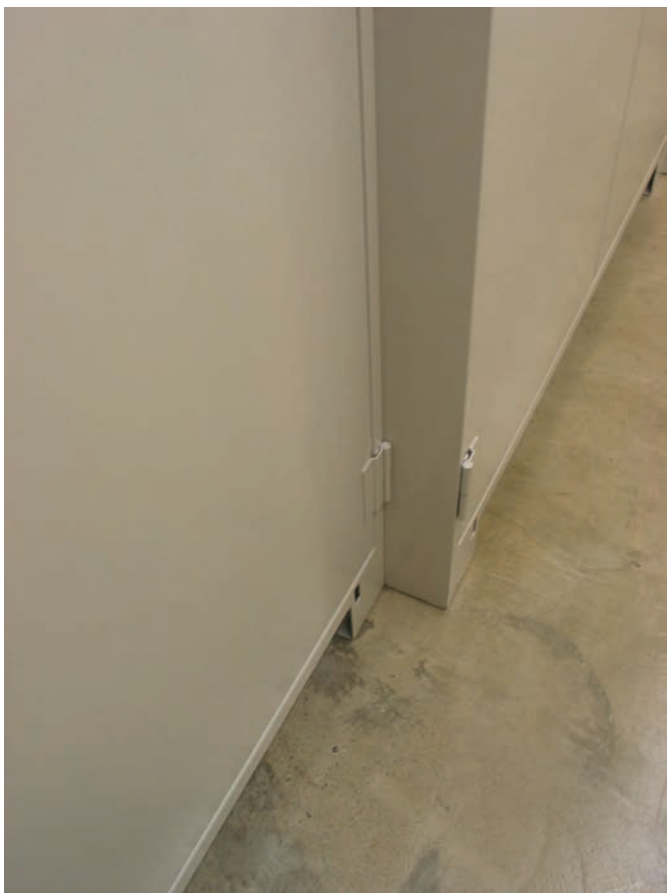
FIGURE 3. Shifting of shelf cabinets, Pod 1, level three. (Smithsonian Institution photo by David Rosenthal.)
