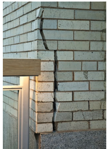
FIGURE 16. Damage to an original 1911 structural beam, basement of Main Building (left) and face brick separated where East Court building connects with Main Building at a bridge walkway (right). (Smithsonian Institution photos by James DiLoreto.)
