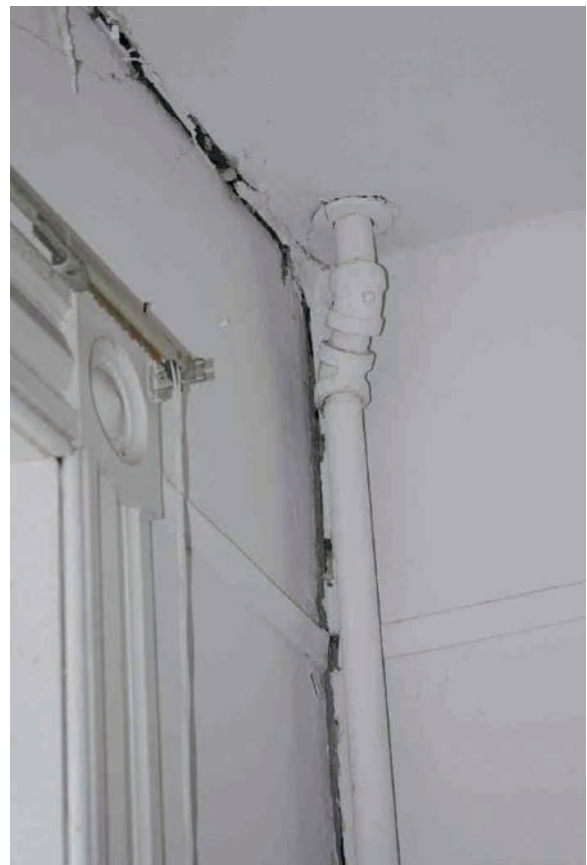
FIGURE 10. Exterior damage from the lateral movement created by the earthquake is seen in the pulling away of the front porch (left). Interior damage resulted in the separation of front and back walls from interior bearing walls and floor framing (right). (Photos by Steve Groh, Smithsonian Institution.)
