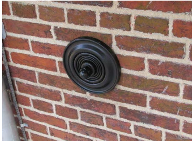
FIGURE 13. In order to tie the floor framing to the exterior walls, the 3 × 10 in (~8 × 26 cm) joists closest to the affected exterior walls were drilled from below to thread new 4 ft (~1 m) long tension rods every 4 ft or so to be anchored by a bolt on one end and a decorative disc plate on the exterior (left). The stainless steel disc has a black baked on finish (right). (Diagram, left: Thornton Tomasetti, Structural Engineers; photo, right: Sharon Park, Smithsonian Institution.)
