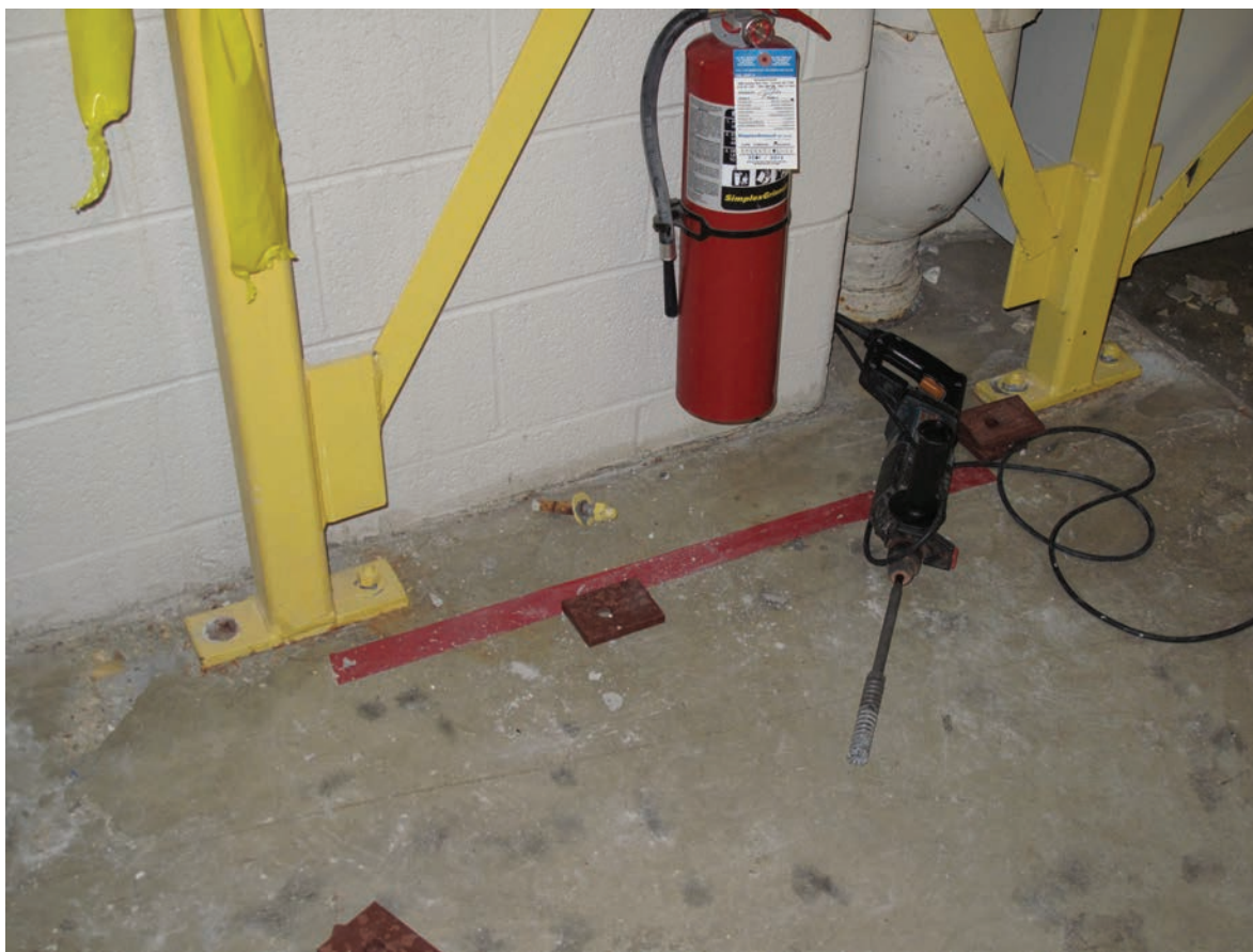
FIGURE 2. Bolts sheared off or torn from Pod 1 floor. (Smithsonian Institution photo by David Rosenthal.)
