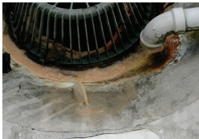
FIGURE 10. Left, typical roof drain in a shallow, membrane-lined basin that may collect rain water and allow it to seep under the membrane; right, a cut was made into the membrane and the water that had collected beneath spurting out. (Photos by Odile Madden.)
