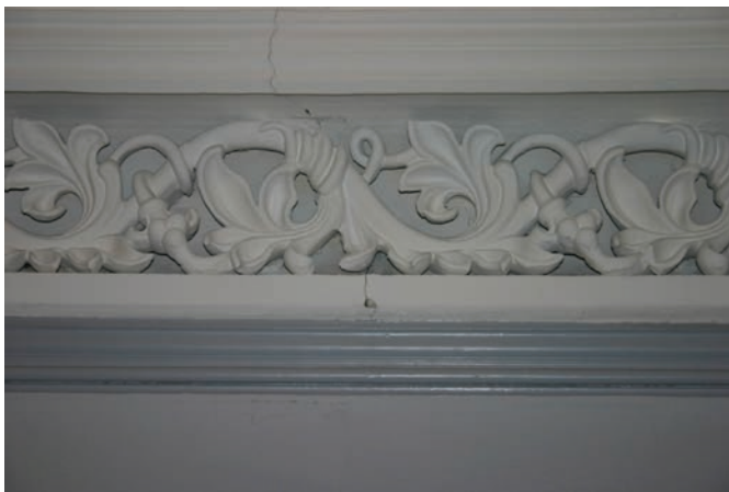
FIGURE 14. The Regent's Conference Room (above) developed a crack (detail, left) that runs through the beam over the bow window. (Smithsonian Institution staff photos.)
