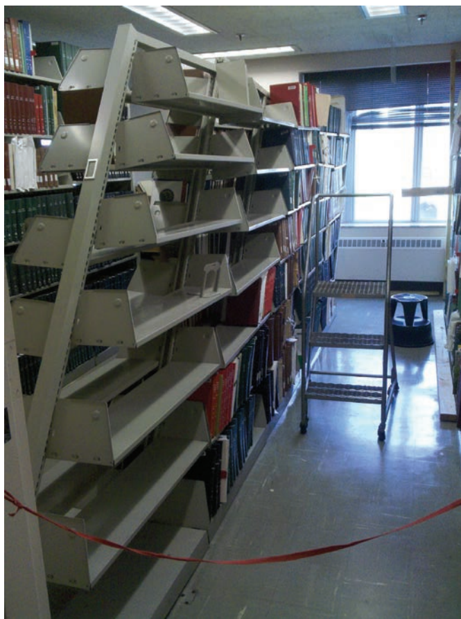
FIGURE 2. Images of twisted and distorted shelving kept in place by the weight of the books. (Smithsonian Institution photos by M. Kalfatovic; see more at http://www.flickr.com/photos/travelinglibrarian/sets/72157627394103839/with/6077290443/ .)
