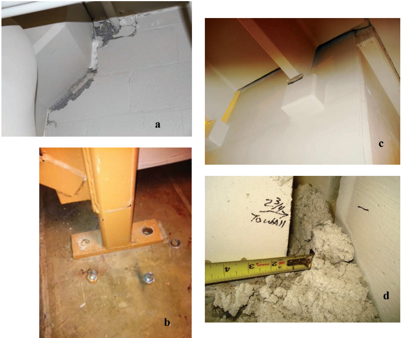
FIGURE 21. Pod 2 damage: (a) cracks along north wall; (b) bolts sheared off from floor; (c) a beam supporting another floor separated from its anchoring; and (d) one of the larger gaps that opened during the earthquake. (Smithsonian Institution photos by Office of Facilities Engineering and Operations staff.)
