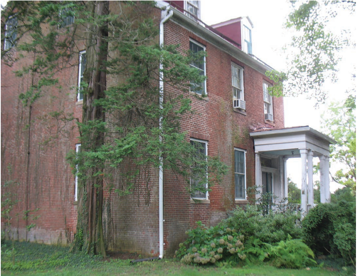
FIGURE 7. Exterior of the 1841 section, shown several months before the earthquake, was stable, but the masonry was in need of repointing as a result of deferred maintenance. This work along with a new standing seam metal roof was in the planning stages but was delayed because of the earthquake. (Photo by David Wright, GWWO, Inc./Architects.)
