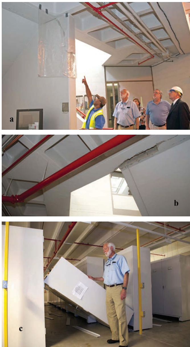
FIGURE 22. (a) G. Wayne Clough (second from left) and others examine a piece cracked off on “street” along Pod 3; (b) major crack along that same street; and (c) Clough examines an empty cabinet toppled over in mezzanine of Pod 1. (Smithsonian Institution photos (a, b) by staff and (c) by James DiLoreto.)
