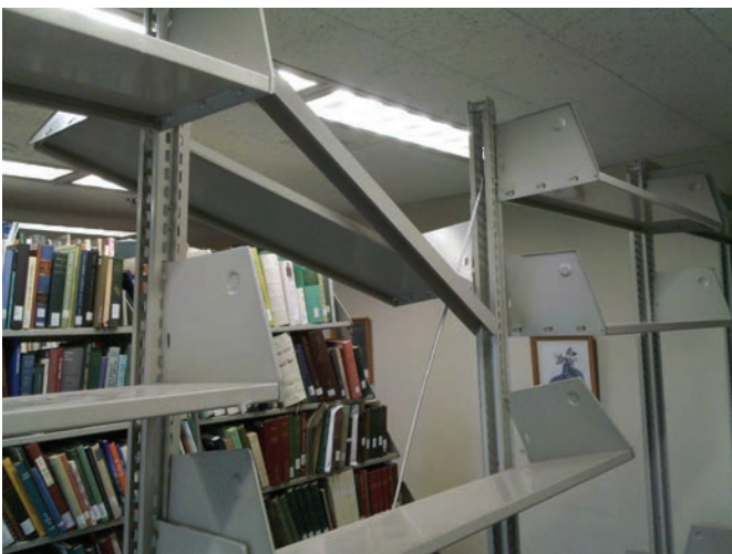
FIGURE 1. Left, twisted and broken shelving. Right, stacks shifted and distorted, leaning perilously against glass windows overlooking Constitution Avenue. (Smithsonian Institution photos by M. Kalfatovic; see more at http://www.flickr.com/photos/travelinglibrarian/sets/72157627394103839/with/6077290443/ .)
