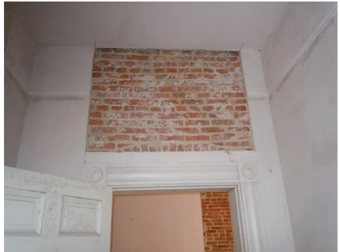
FIGURE 14. Images, once plaster was removed, show the diagonal cracks over a doorway before (left) and after (right) repointing. As with other interior repairs, the plaster will be replaced at a later date. (Smithsonian Institution staff photos.)
