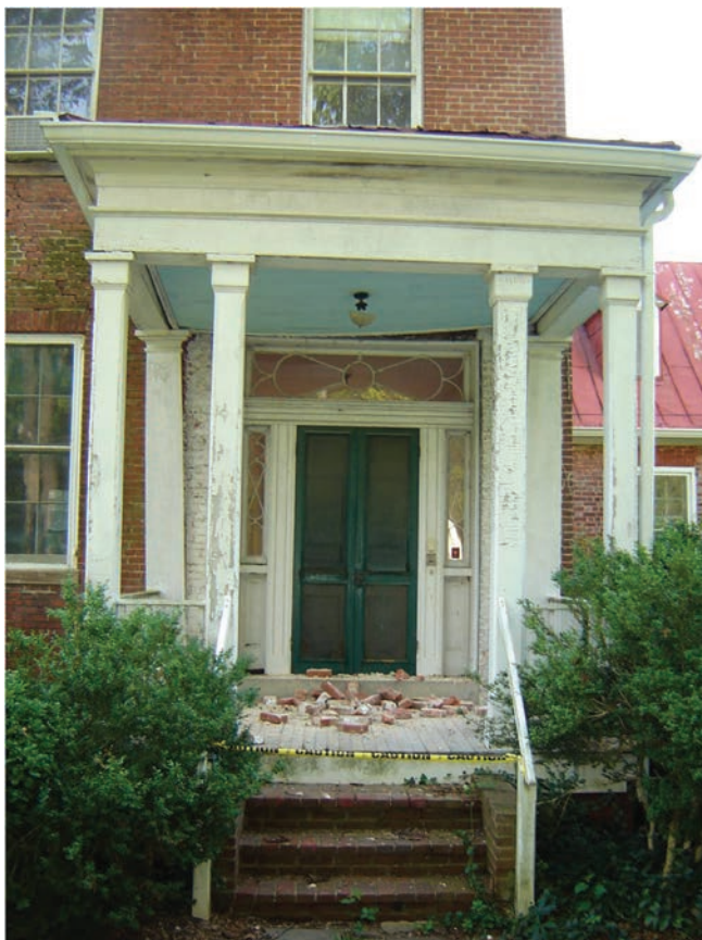
FIGURE 10. Exterior damage from the lateral movement created by the earthquake is seen in the pulling away of the front porch (left). Interior damage resulted in the separation of front and back walls from interior bearing walls and floor framing (right). (Photos by Steve Groh, Smithsonian Institution.)
