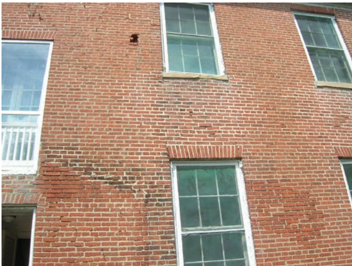
FIGURE 9. The exterior and interior of the 1841 section had suffered from deferred maintenance while the house was in a life tenancy situation. The exterior brickwork (left) was in need of repointing; and the basement (right) had a number of temporary bracing supports, which luckily kept the house from having major structural damage during the earthquake. (Photos by David Wright, GWWO, Inc./Architects.)
