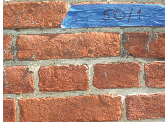
FIGURE 15. The image on the left shows the two eras of brick and mortar work. Mock-ups were developed to test for specific composition and appearance to match each era. On the right is seen a sample for the 1841 section with the bottom two courses of new lime-rich mortar with shell aggregate to match the upper course by the blue tape. The 1735 section had a slightly different aggregate mix and a tooled joint detail. (Photos: left, Raymond Jones, Smithsonian Institution; right, Bryan Fisher, GWWO, Inc./Architects.)
