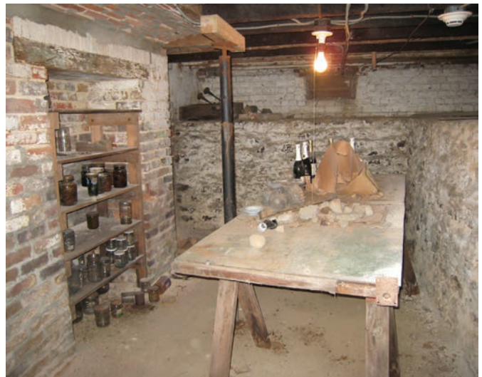
FIGURE 9. The exterior and interior of the 1841 section had suffered from deferred maintenance while the house was in a life tenancy situation. The exterior brickwork (left) was in need of repointing; and the basement (right) had a number of temporary bracing supports, which luckily kept the house from having major structural damage during the earthquake. (Photos by David Wright, GWWO, Inc./Architects.)
