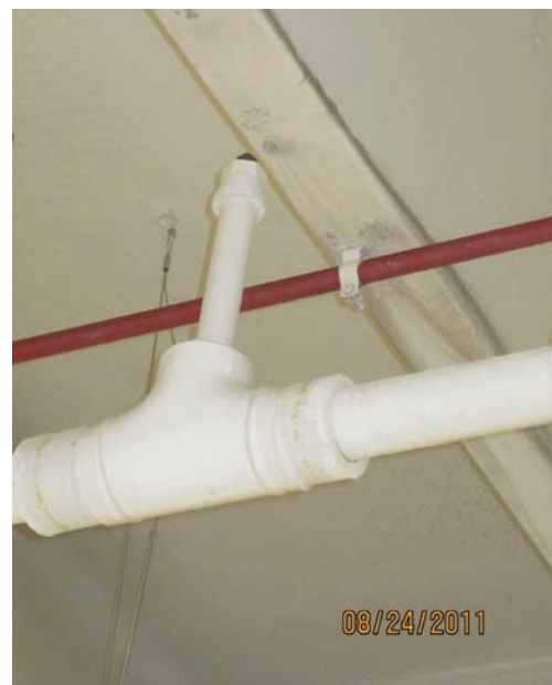
FIGURE 3. Above, sprinkler head as installed; right, sprinkler head in Pod 3 sheared off during the earthquake. (Smithsonian Institution photo by Catharine Hawks, NMNH.)
