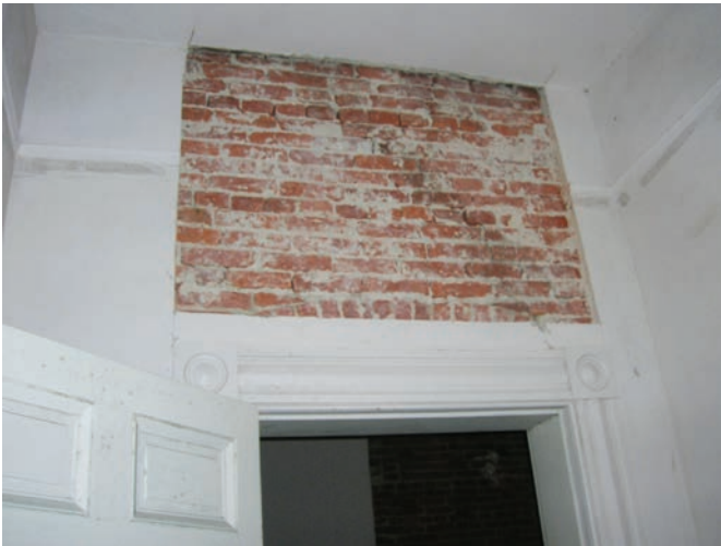
FIGURE 14. Images, once plaster was removed, show the diagonal cracks over a doorway before (left) and after (right) repointing. As with other interior repairs, the plaster will be replaced at a later date. (Smithsonian Institution staff photos.)
