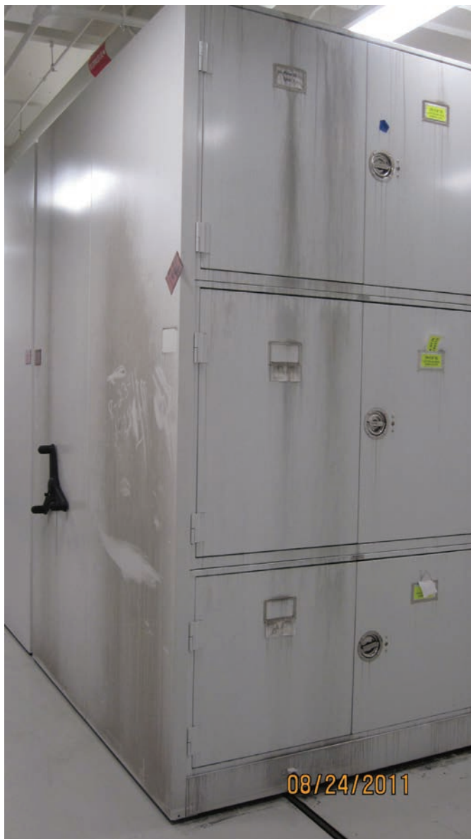
FIGURE 4. Cabinets stained by the blackish water released from the broken sprinkler heads in Pod 3. (Smithsonian Institution photo by Catharine Hawks, NMNH.)
