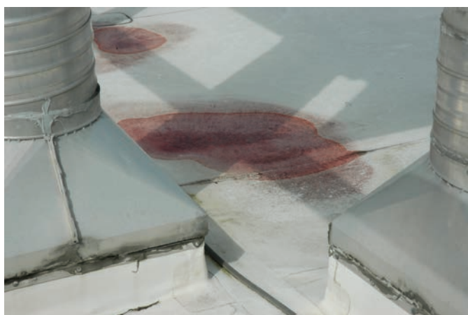
FIGURE 9. Red staining in standing water presumably resulting from microorganism growth. (Smithsonian Institution photo by Carol A. Grissom, MCI.)
