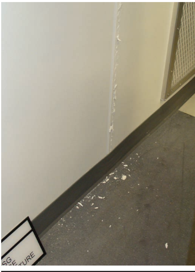
FIGURE 1. Cracks in the wall of Pod 3 at the MSC. (Smithsonian Institution staff photo.)
