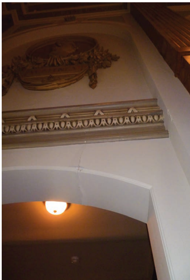
FIGURE 19. Cracks in the Luce Center of the Smithsonian American Art Museum, 26 August 2011 (Smithsonian Institution photo by James DiLoretto).
