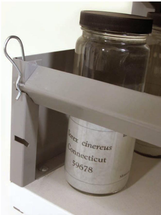
FIGURE 4. Earthquake bars were originally designed to slide into slats on each side of every shelf. Hairpin cotter pins were applied to fasten the bars into place and prevent future failure. (Photos by Suzanne C. Peurach, USGS Patuxent Wildlife Research Center.)
