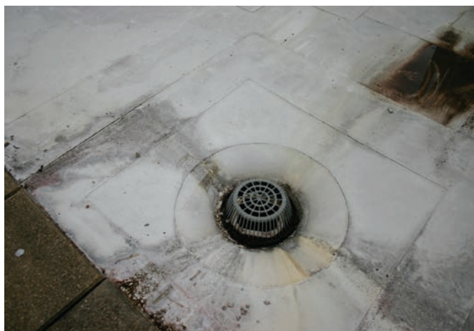
FIGURE 10. Left, typical roof drain in a shallow, membrane-lined basin that may collect rain water and allow it to seep under the membrane; right, a cut was made into the membrane and the water that had collected beneath spurting out. (Photos by Odile Madden.)
