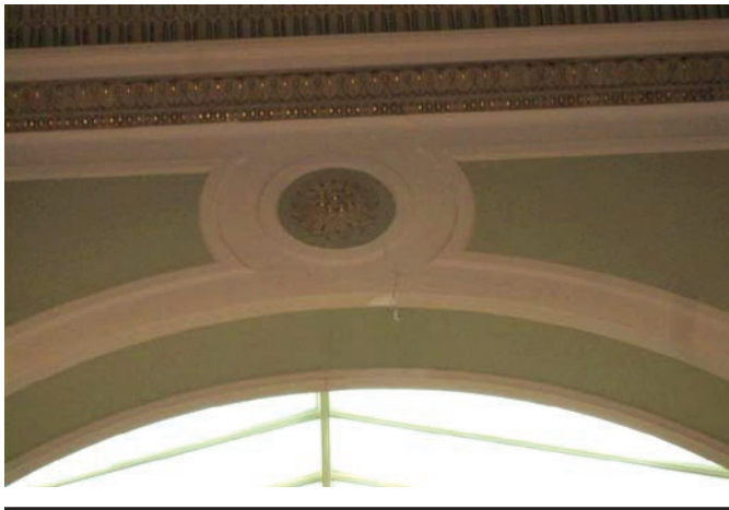
FIGURE 1. One of several cracks in the arches around the Great Hall (above) and its pilasters (right). (Smithsonian Institution photos by Office of Facilities, Management and Reliability staff.)
