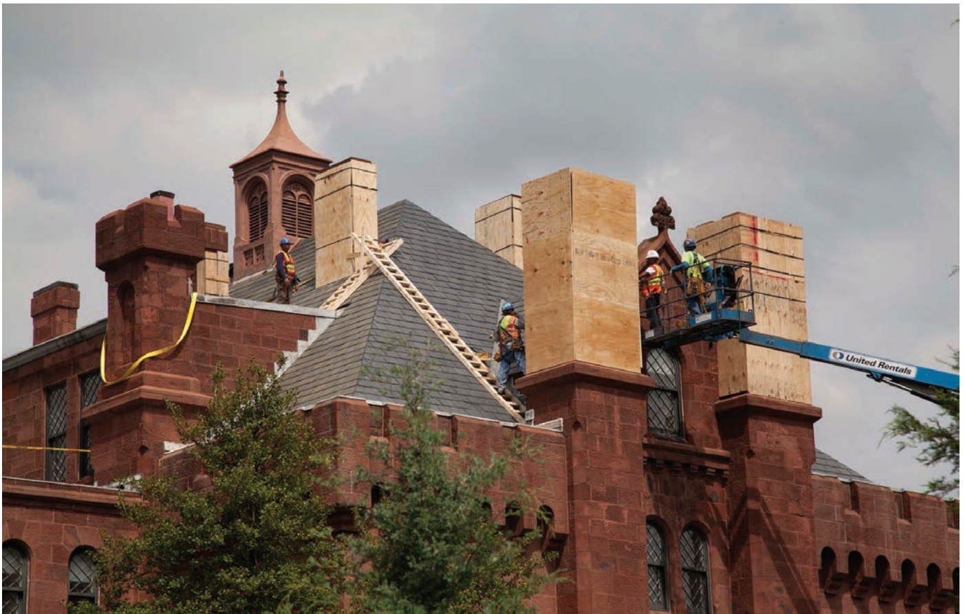
FIGURE 13. Stabilization of damaged stonework underway on 26 August 2011. (Smithsonian Institution photo by Eric Long.)
