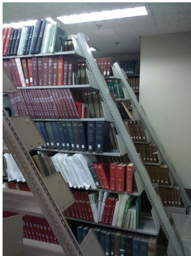
FIGURE 2. Images of twisted and distorted shelving kept in place by the weight of the books. (Smithsonian Institution photos by M. Kalfatovic; see more at http://www.flickr.com/photos/travelinglibrarian/sets/72157627394103839/with/6077290443/ .)
