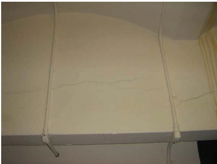
FIGURE 16. Damage to an original 1911 structural beam, basement of Main Building (left) and face brick separated where East Court building connects with Main Building at a bridge walkway (right). (Smithsonian Institution photos by James DiLoreto.)
