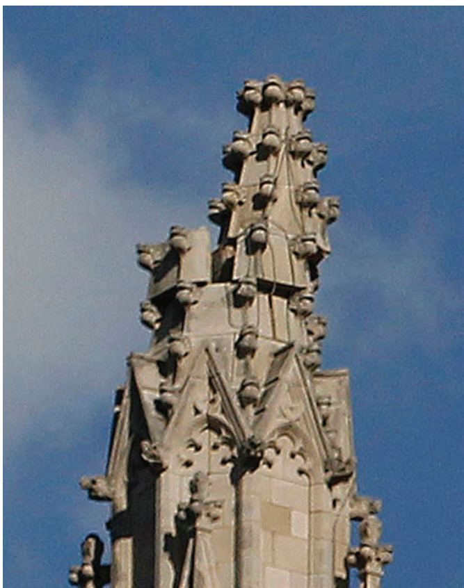
FIGURE 9. The National Cathedral in August 2008 and detail of damage it suffered in August 2011 during the largest earthquake to hit the region in more than 100 years. Note that long and spiky objects tend to suffer more—three of the four high spires at the top of the cathedral were damaged. (Photos: Cathedral, courtesy NCinDC, http://www.flickr.com/photos/ncindc/2794096753 ; spire detail, REUTERS, Jason Reed.)
