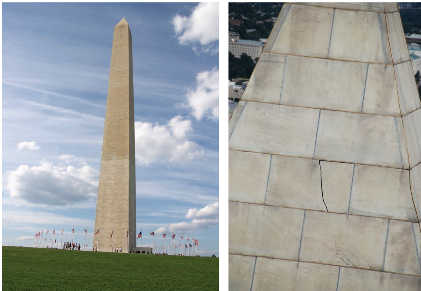
FIGURE 10. The Washington Monument in September 2005 (left) and detail of the crack that developed across one block on the pyramidion during the August 2011 earthquake (right). (Photos: left, courtesy Corey L. Kliever, Washington, D.C., Convention and Tourism Corporation, www.washington.org [ http://www.flickr.com/photos/wctc/79492470 ]; right, National Park Service.)
